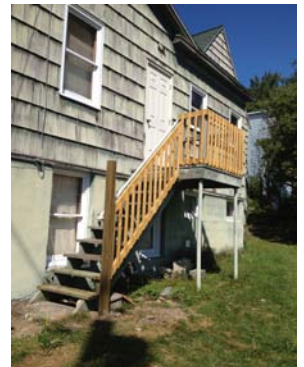
Repair stairs in Groton, NY
